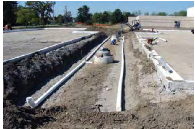
Underdrain in trench
