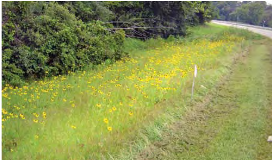
Vegetated filter strip along roadway
