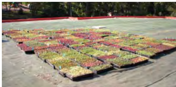
Plugs prior to planting extensive vegetated roof
