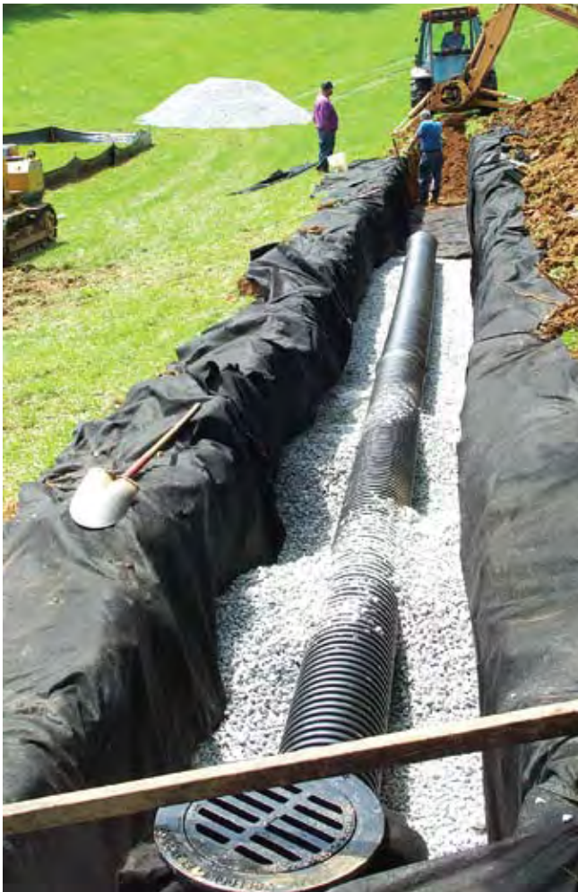
Infiltration trench with geotextile
