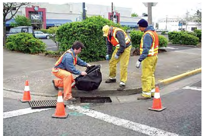
Installing a bag type catch basin insert
