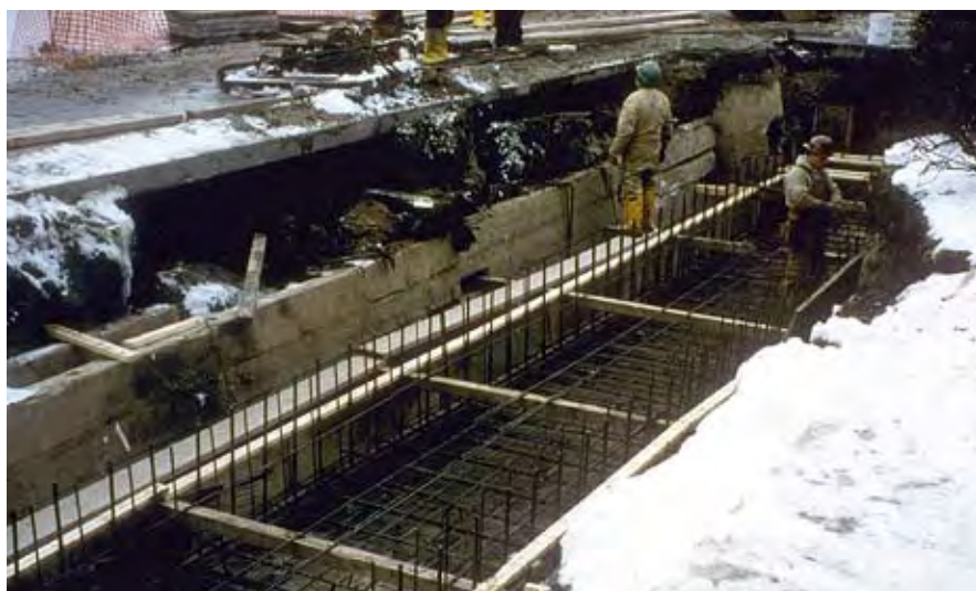
Installation of a sand filter
