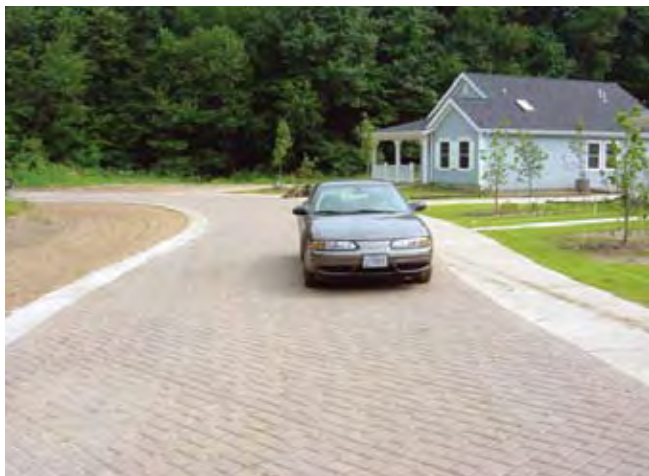
Permeable paver street in Dowagiac, MI
