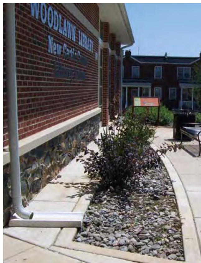
Example of Infiltration Planter Box
