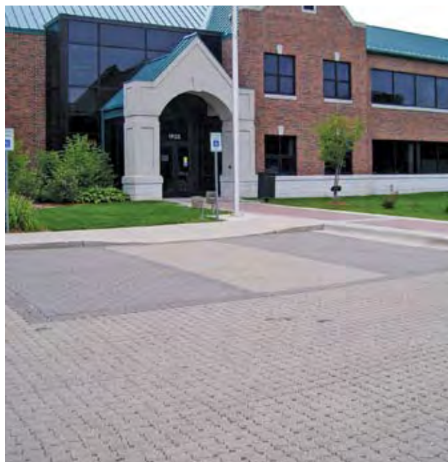
Permeable paver lot at Grand Rapids Environmental Services Building
