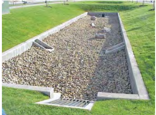
Surface contained filter
