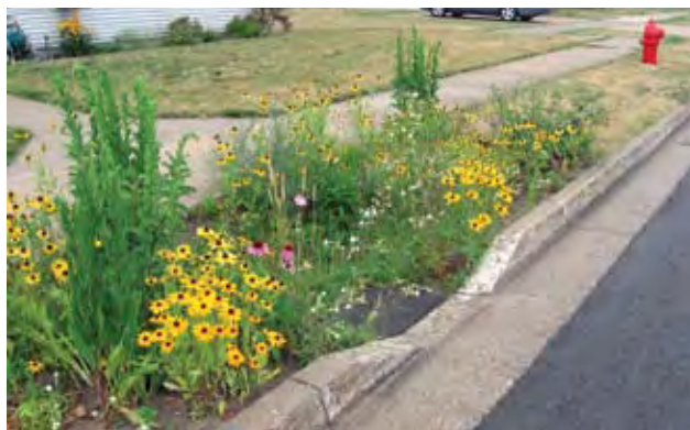
Curb cut into bioretention area/rain garden
