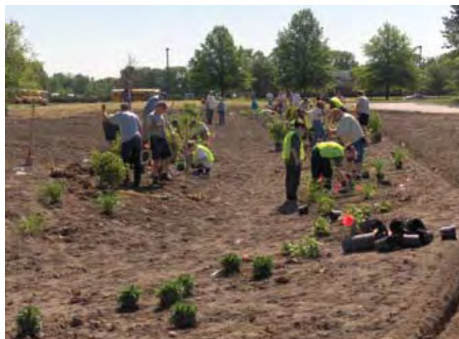
Installing bioswale vegetation at Macomb County Public Works Office.
