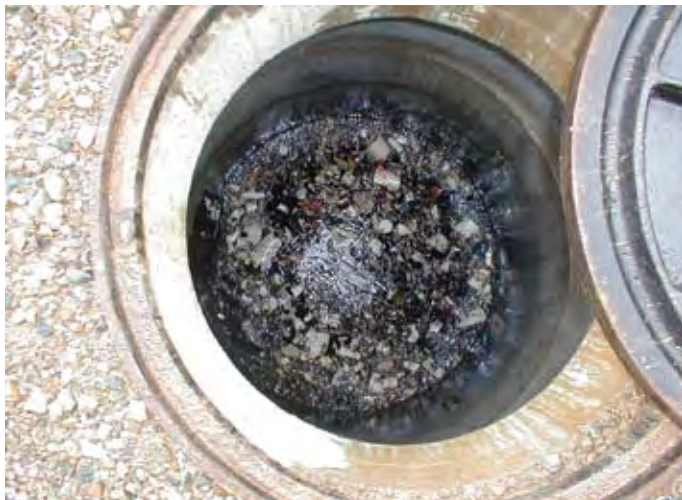
Screening vortex device with floating debris
