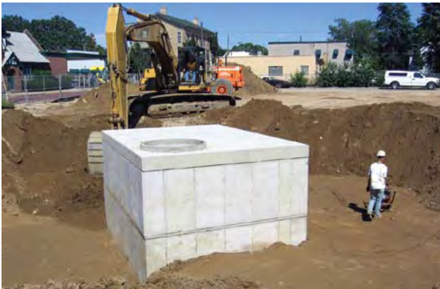
Underground cistern tank
