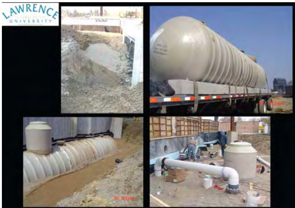
Underground cistern at Lawrence Technological University
