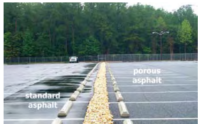
Figure 7.33 Riverstone edge serves as a backup inlet into the infiltration bed under the porous asphalt
