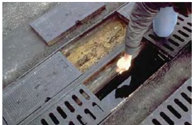
Linear perimeter filter in trench drain
